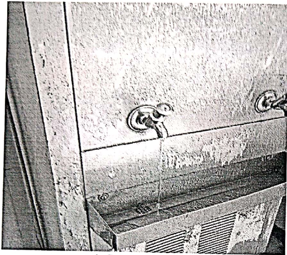
1. Leakage of Tap
