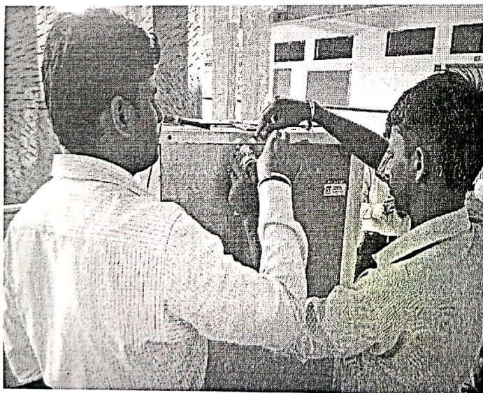
3. Removing dust and old Teflon tap from connector
