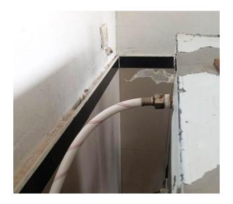
1. Leakage of Tube
